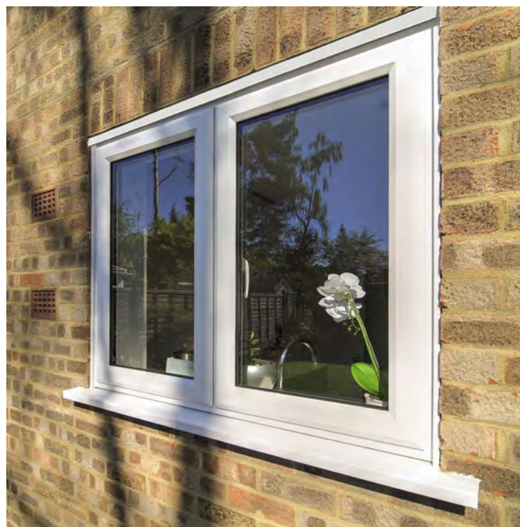
Concealed Ventilation installed through the outer frame
