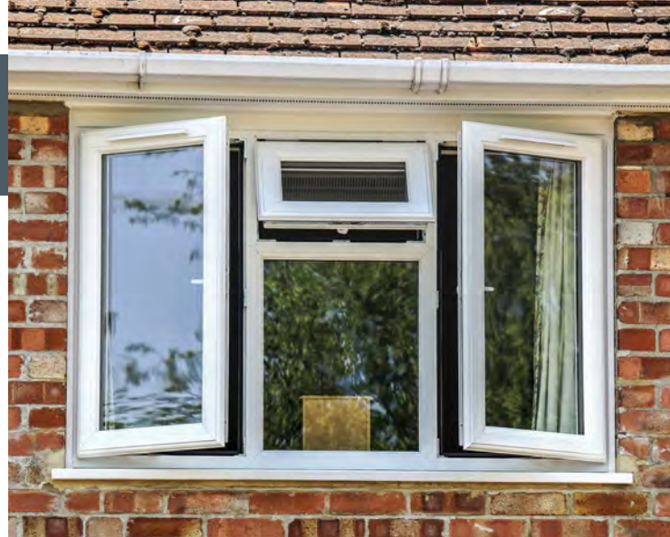
Trickle Vents installed through the window sashes
