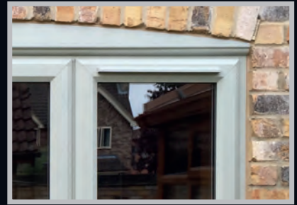
Trickle vent through a Rebated Sash
